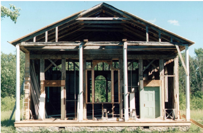
The removal of a false wall and wall coverings behind the stage exposed the full palladian window. Removing the false ceiling revealed the arched side windows and the top of the palladian window behind the stage. Also visible is the original expanded wood lath of the side walls. The excavated space housing the kitchen below the stage is just visible, as is its access door to the right.
