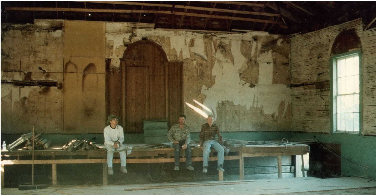
The removal of a false wall and wall coverings behind the stage exposed the full palladian window. Removing the false ceiling revealed the arched side windows and the top of the palladian window behind the stage. Also visible is the original expanded wood lath of the side walls. The excavated space housing the kitchen below the stage is just visible, as is its access door to the right.
