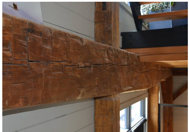
Tapered Swing Beam Installed Upside Down in the L&A Mutual Insurance Office
