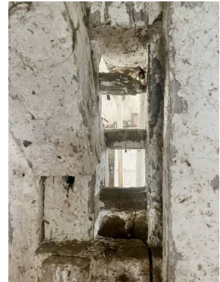
Mortise where the swing beam once fit
