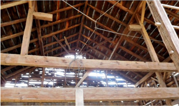
Tie Beam Cut Off
