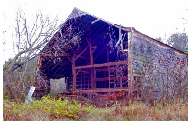
Collapsed East Wall
