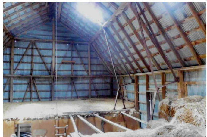
Mow area showing metal trusses
